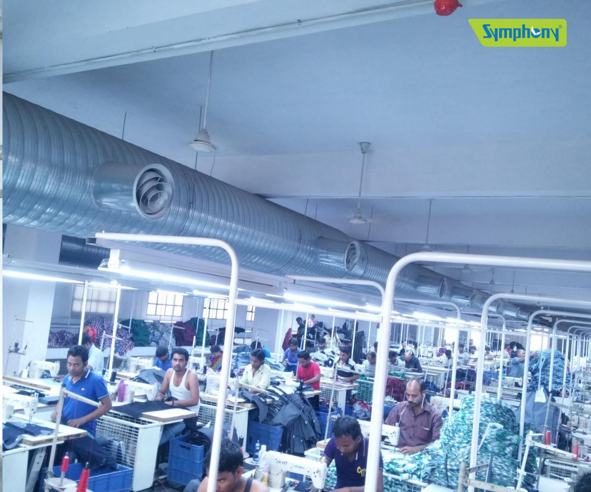
Ducting – All machines are connected to 140 feet duct having 28 jet diffusers.
