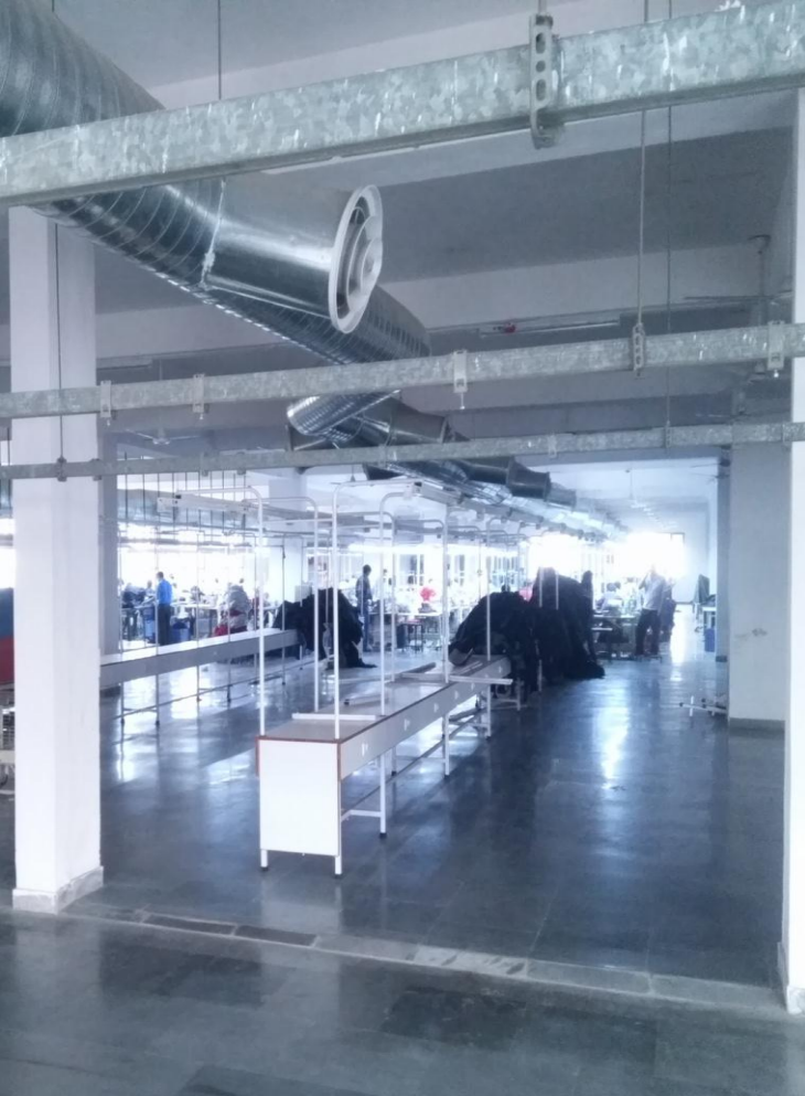
Ducting – All machines are connected to 140 feet duct having 28 jet diffusers.
