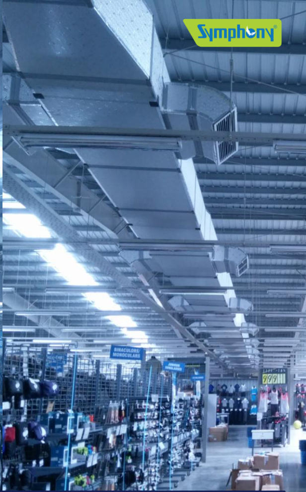
Ducting – All machines are connected to 150 feet duct having 20 outlets.
