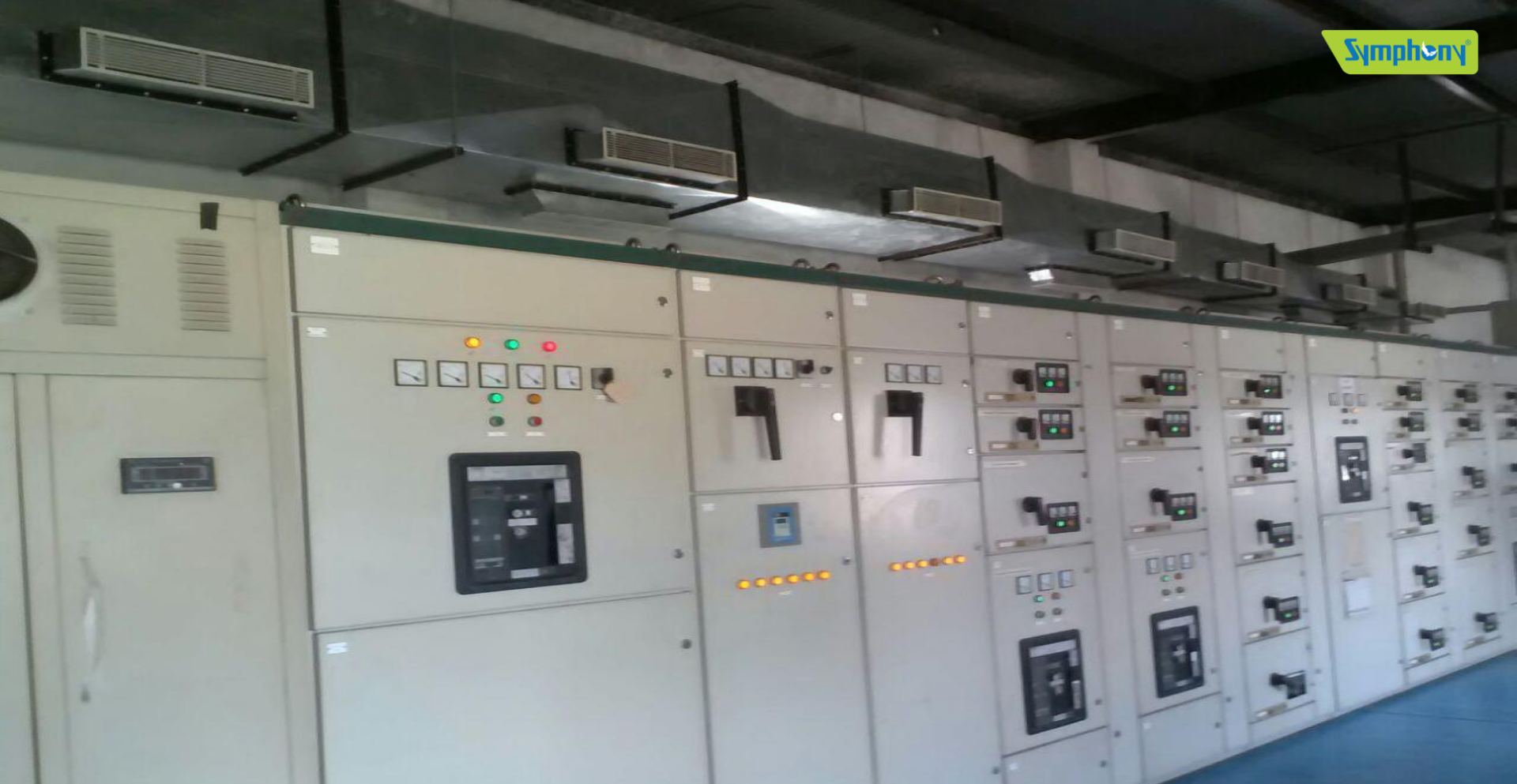
Ducting – Machine is connected to 62 feet duct having 13 outlets.
