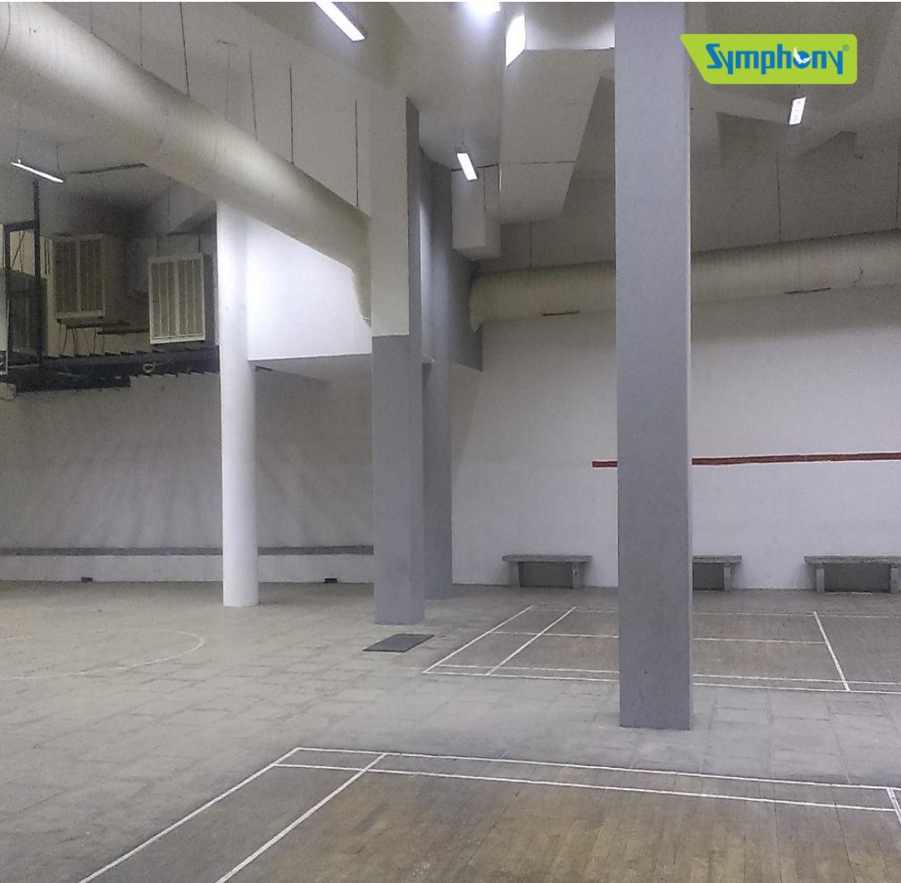
Ducting – All machines are connected to 80 feet duct having 12 outlets.
