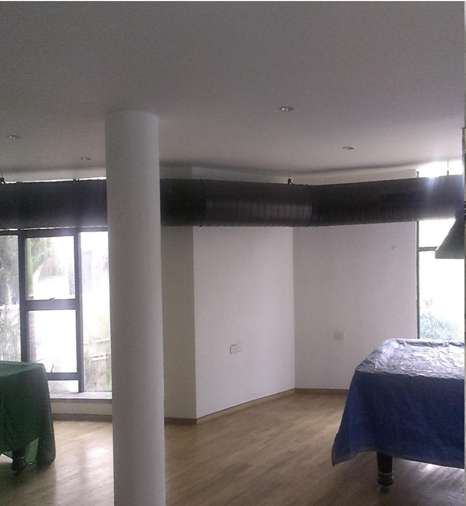
Ducting – All machines are connected to 80 feet duct having 12 outlets.
