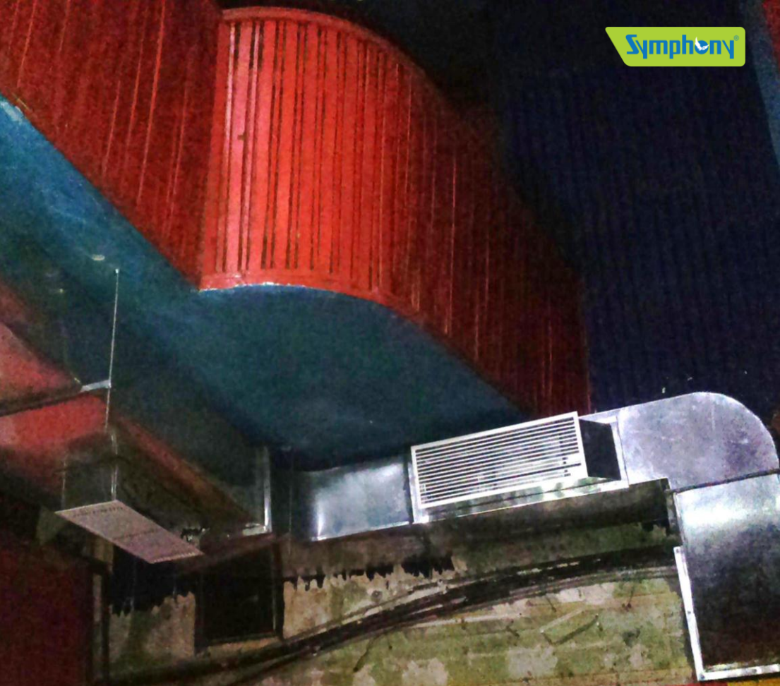
Ducting – 8 machines are connected to direct outlet grill & 4 machines are connected to 45 feet duct having 3 outlets.
