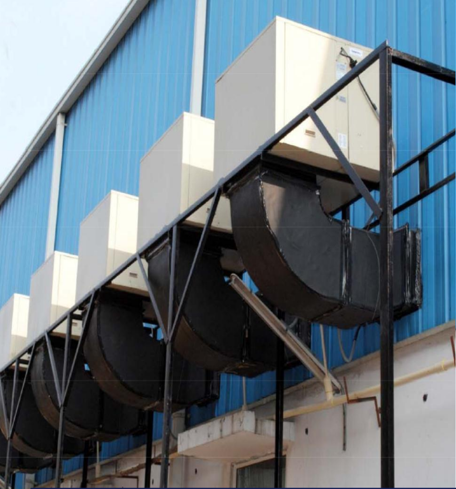
Ducting – All machines are connected to direct outlets grill.
