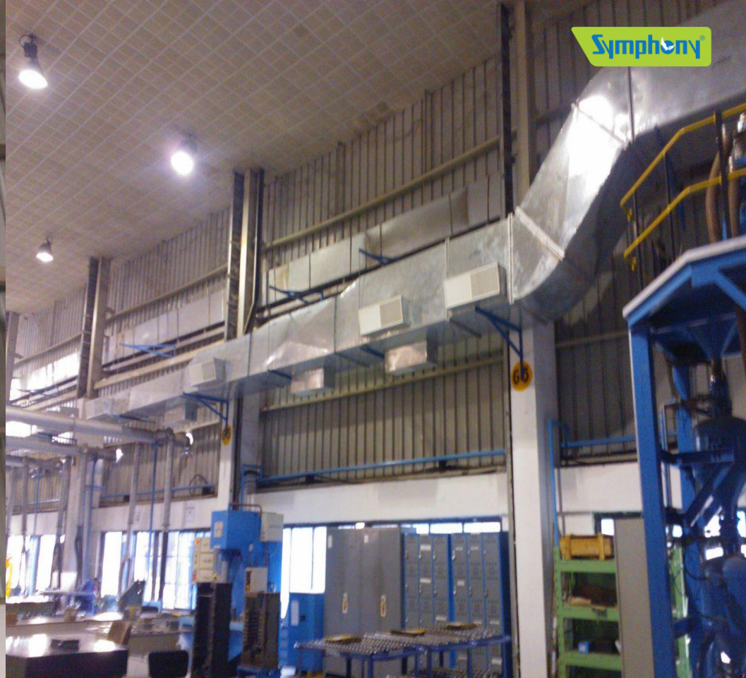
Ducting – 12 machines are connected to 15 feet duct with plenum having 12 jet diffusers & 3 machines are connected to 120 feet duct having 9 outlets.
