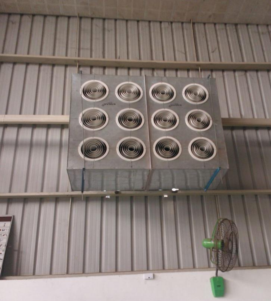
Ducting – 12 machines are connected to 15 feet duct with plenum having 12 jet diffusers & 3 machines are connected to 120 feet duct having 9 outlets.
