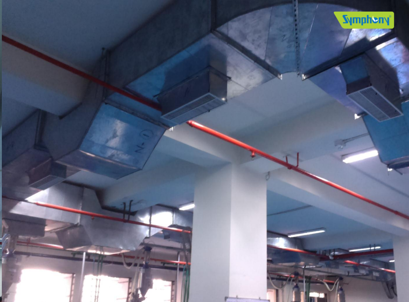
Ducting – Machine is connected to 90 feet duct having 14 outlets.
