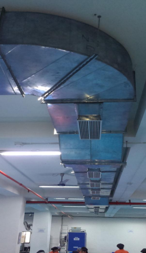
Ducting – Machine is connected to 90 feet duct having 14 outlets.
