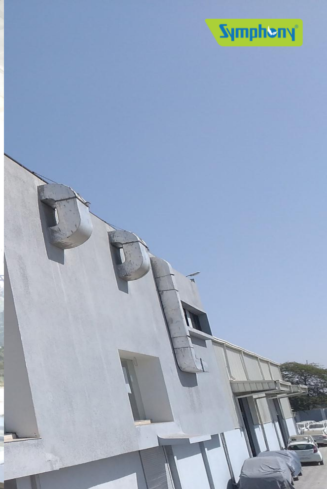
Ducting – All machines are connected to 40 feet duct having 1 to 2 outlets.
