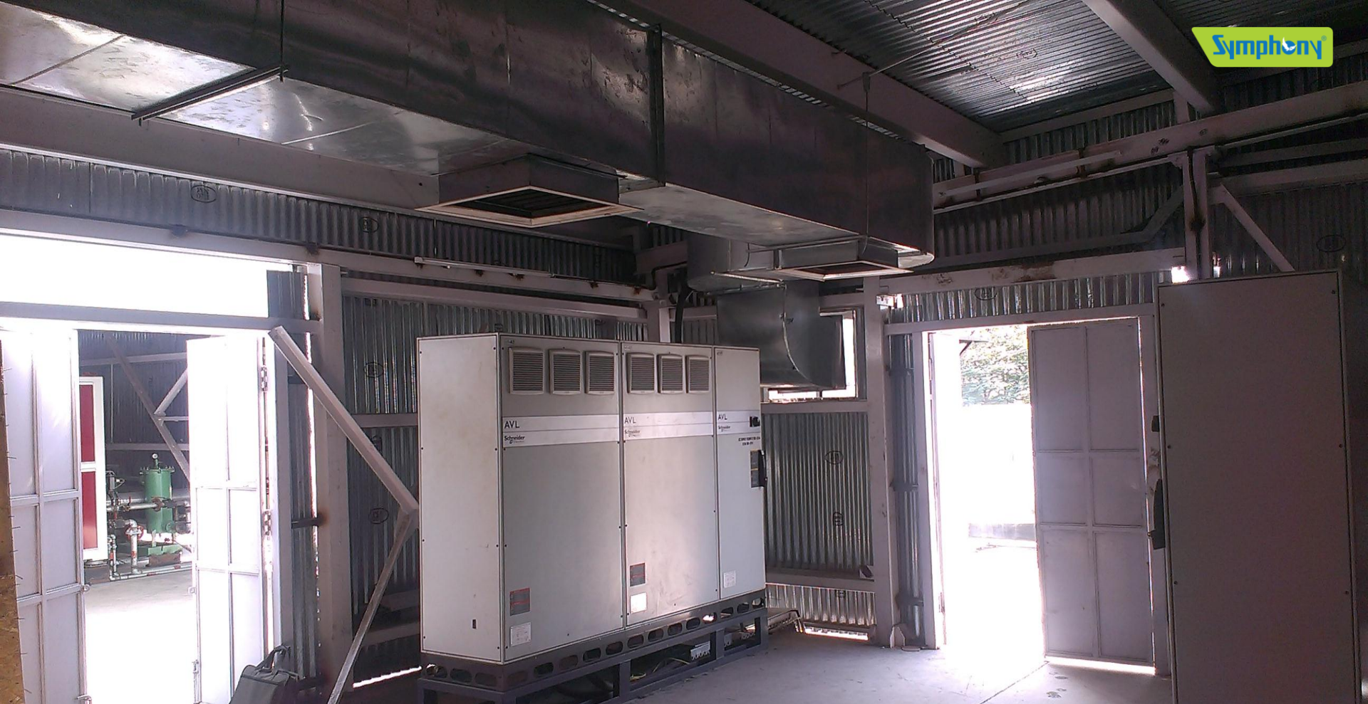
Ducting – Machine is connected to 40 feet duct having 3 outlets.
