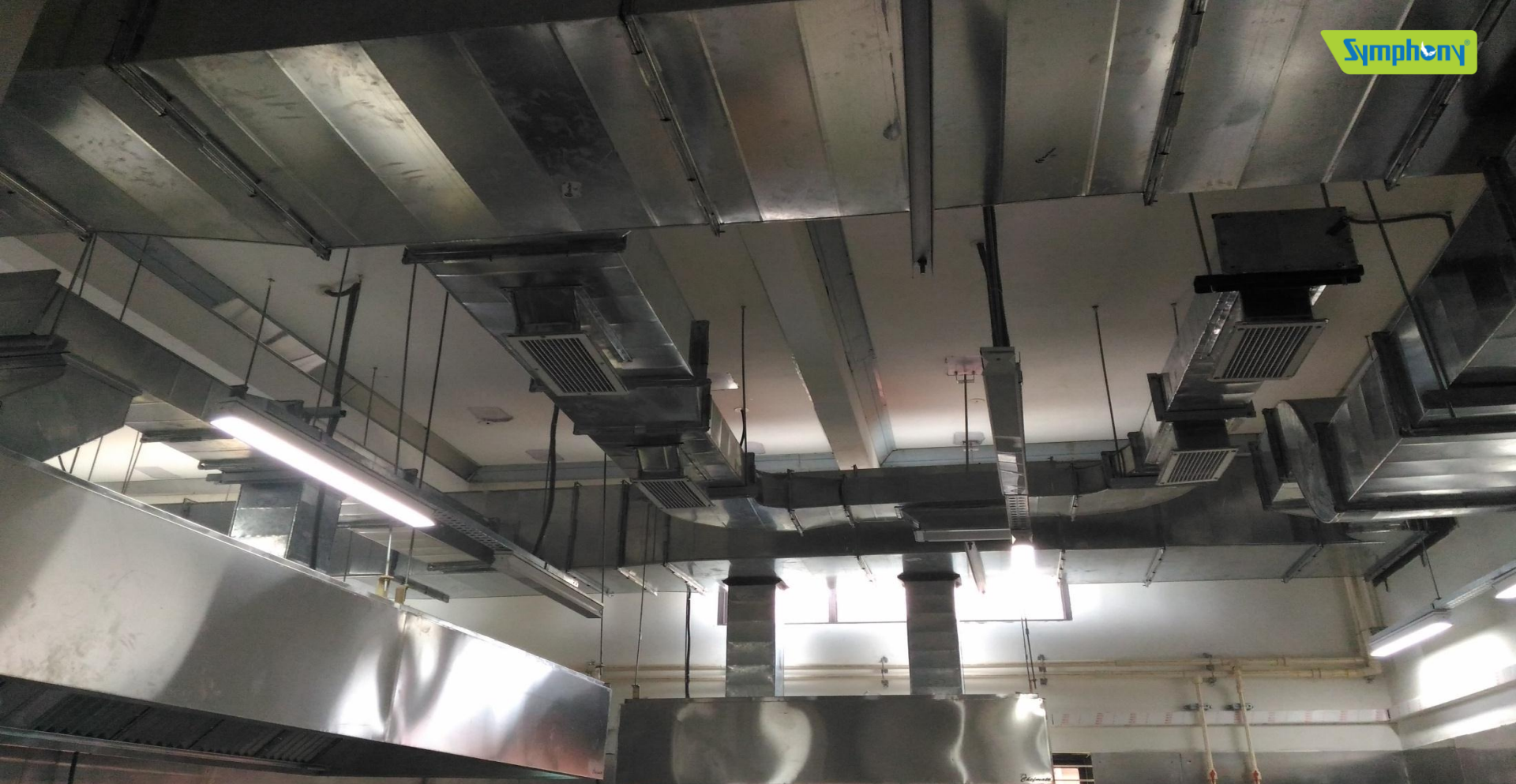
Ducting – Machine is connected to 120 feet duct having 18 outlets.
