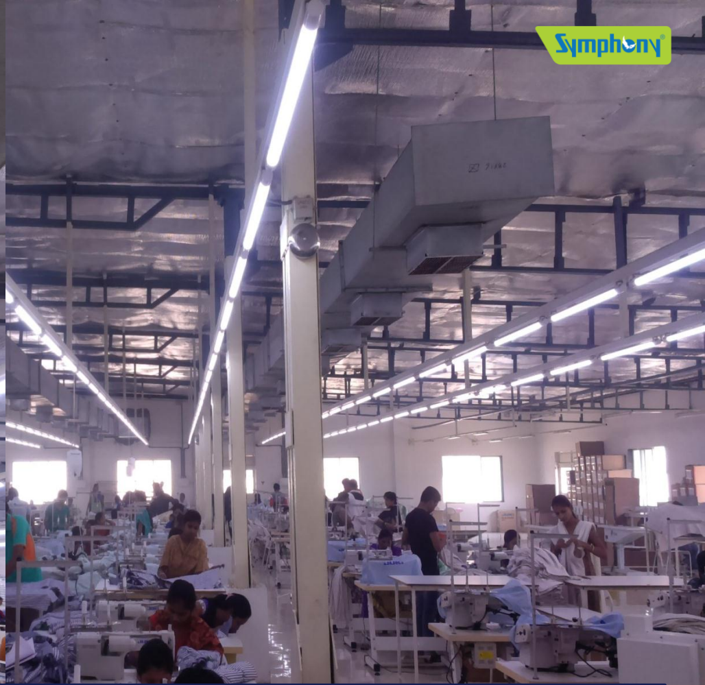
Ducting – All machines are connected to 100 feet duct having 12 outlets.
