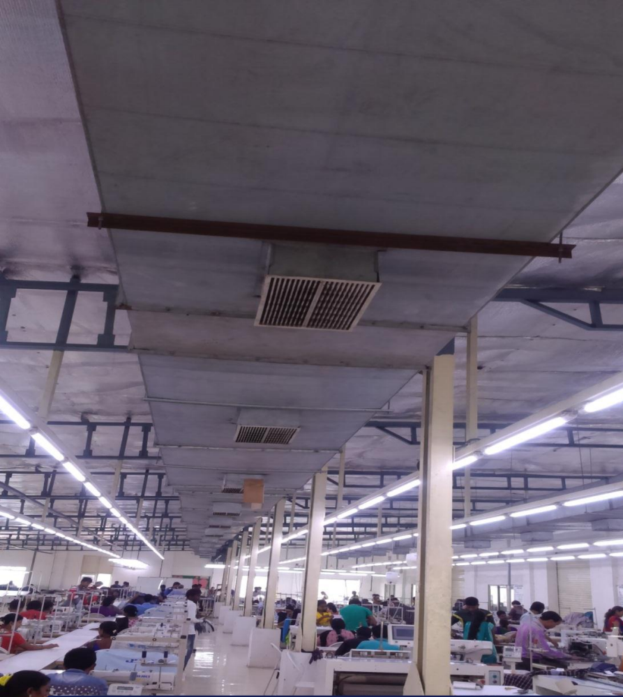
Ducting – All machines are connected to 100 feet duct having 12 outlets.
